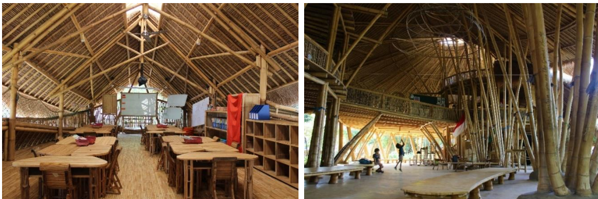
Figure 3. A classroom, and the 'Heart of School' at Green School Bali: a six-storey building constructed entirely from round-pole bamboo. Credit: INBAR.
